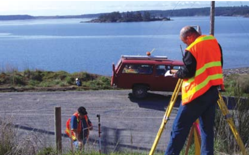
▲ County employees conduct ground control survey in support of the 2008 orthophotography project.
